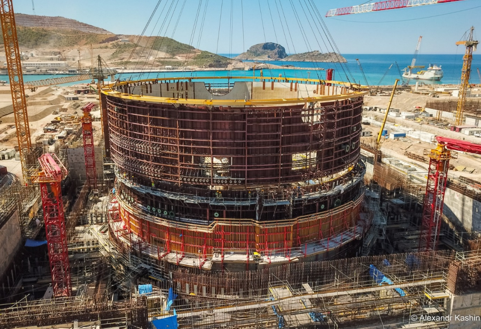
Fig. 4 – Akkuyu nuclear powerplant under construction. Source: http://www.akkuyu.com/third-tier-of-the-internal-containment-installed-at-akkuyu-npp-unit-1
