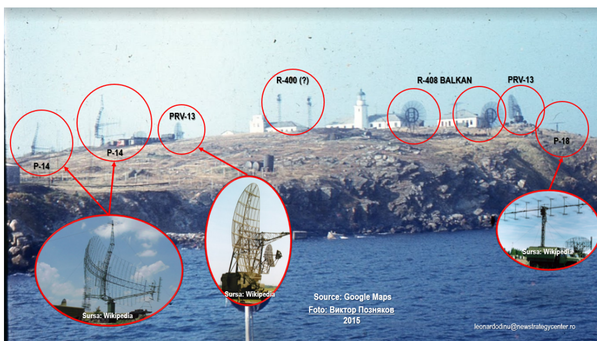
Fig. 8. Radar systems deployed on the island. Source: Google Maps; Wikipedia (footnote 15, 16, 18); New Strategy Center.
